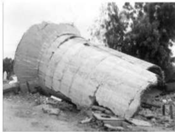
Fig. 1 Collapse of water tank in Bhuj
